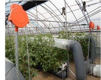
Heating duct (moving up and down)
