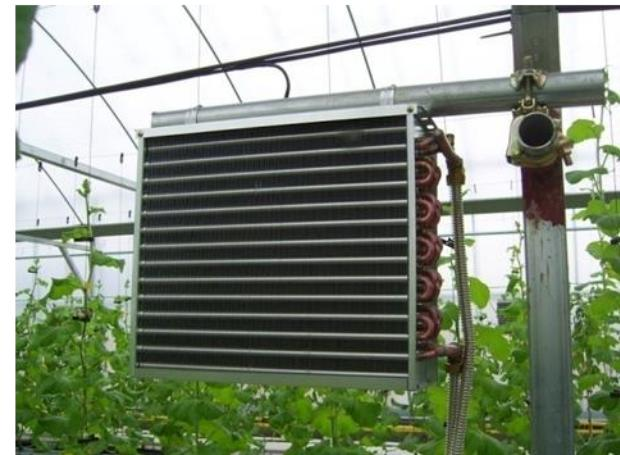
Cooling and heating by fan coil unit
